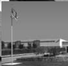
McKinney data centre, Texas.
