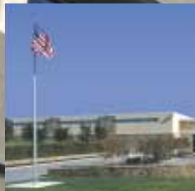
McKinney data centre, Texas.
